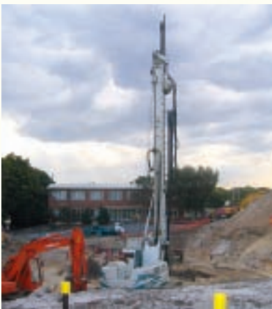
Firm foundations, the laying of the piles for the new building.
