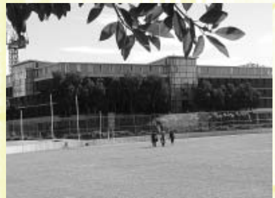
The refurbished building viewed from the Village Green.
