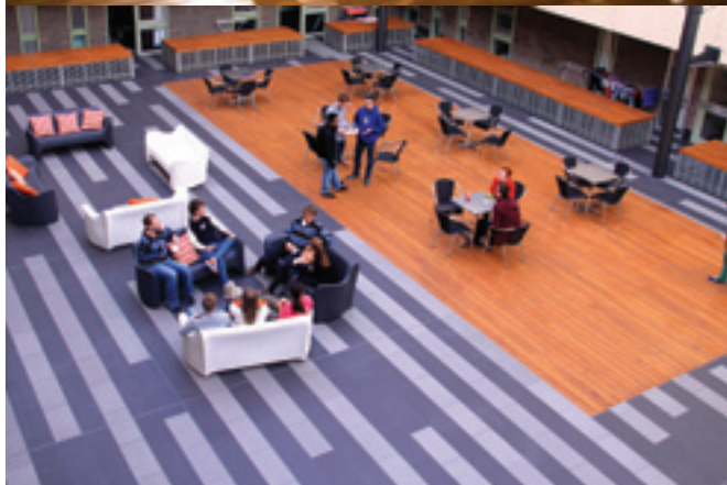
The water damage issue has finally been resolved. A glass and polycarbonate roof has been placed over the courtyard. A system of louvres and vents has been engineered to naturally regulate the temperature inside and keep the rain out. The courtyard is now an all-weather, multi-purpose facility for collegians.
