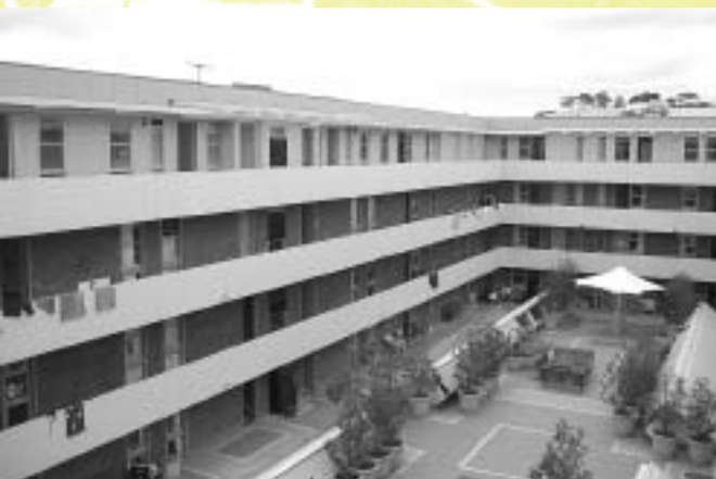
The fourth floor goes up at New College. Photo by Trevor Cairney.
