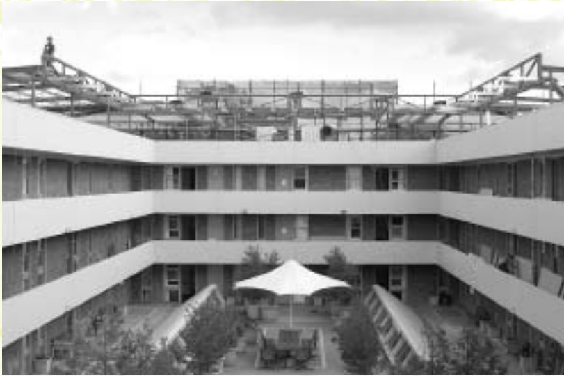
View of construction from the courtyard. Photo by Paul Doak.
