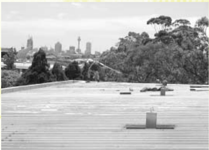
Third-floor roof prior to construction. Photo by Paul Doak.
